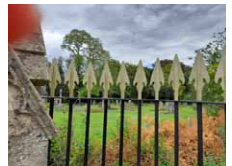
The newly painted railings
